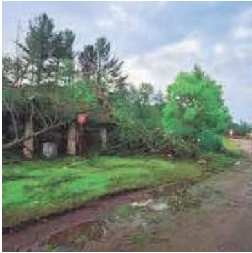
Tornado damage, July 2025, Menominee Co CFZ Office
